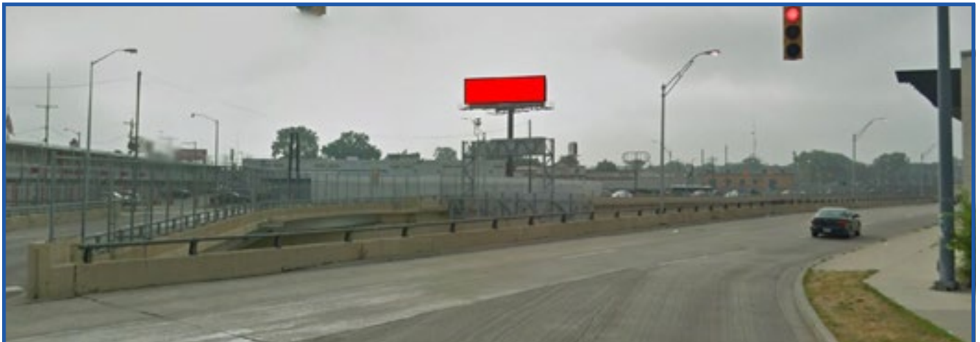
View: Lodge Fwy Service Dr. South
