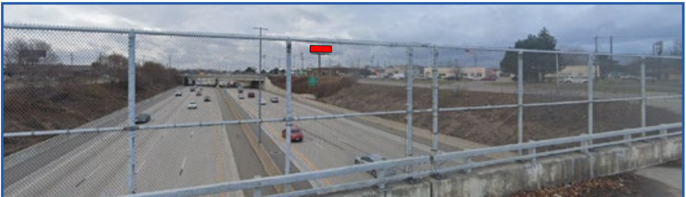
I-696 EB overpass to I-696 WB service drive
